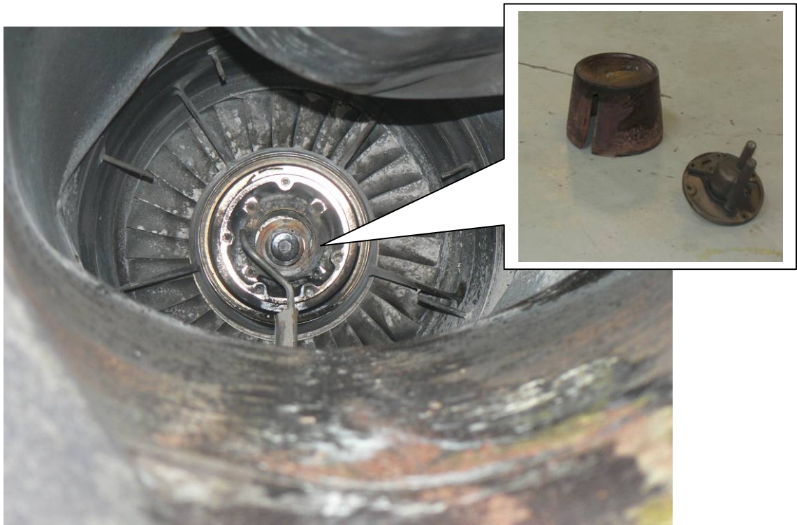
Figure 7; The right-hand engine with rear bearing cover and tail cone missing. The insert picture shows similar parts from another engine.
